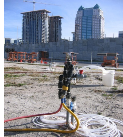
Full-Scale Injection in Downtown Orlando
